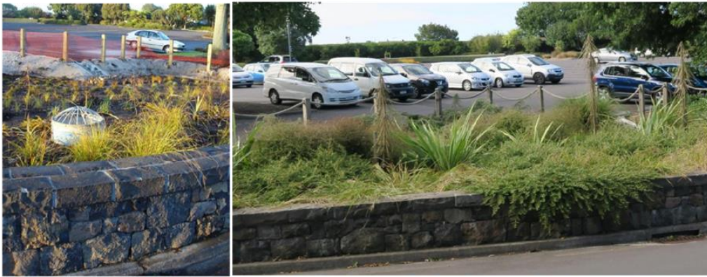
Raingarden treating parking lot runoff shortly after planting, showing the overflow, and after about three years; a diverse range of native groundcovers is used including coprosmas, shrubby pohuehue, sedges and Astelia, with lancewood providing interest.
