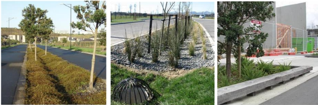
A 50 to 100 mm drop over concrete allows sheet flow into these swales planted with scrambling pohuehue and pohutukawa trees (left, Auckland), low sedges and taller rushes with kōwhai and ribbonwood trees (centre, Lincoln, Canterbury) and mountain flax and pohutukawa (right, Waitakere).
