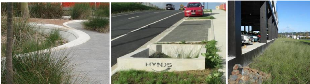
Edge details are important. Left – raised edges with colour differentiation from the pavement reduce risk of pram and pedestrian entry in this public space (Adelaide Zoo); centre – tall concrete edge creates car and cyclist hazard, and high-maintenance grass strip between footpath and device (Auckland); right – sharp drop, colour contrast and bollards along edge of large raingarden that receives runoff from downpipe (with boulders to dissipate energy)
