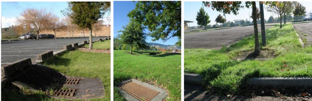
Physical protection and effective drop into a grass swale planted with totara (Manukau), trees should be planted on the sides of a swale as shown in Saxton Fields (centre). Trees should not be planted in the centre of swales as 1) the surface rises with tree age 2) bare sprayed areas around tree bases should not be in the main flow path (right, Stoke).
