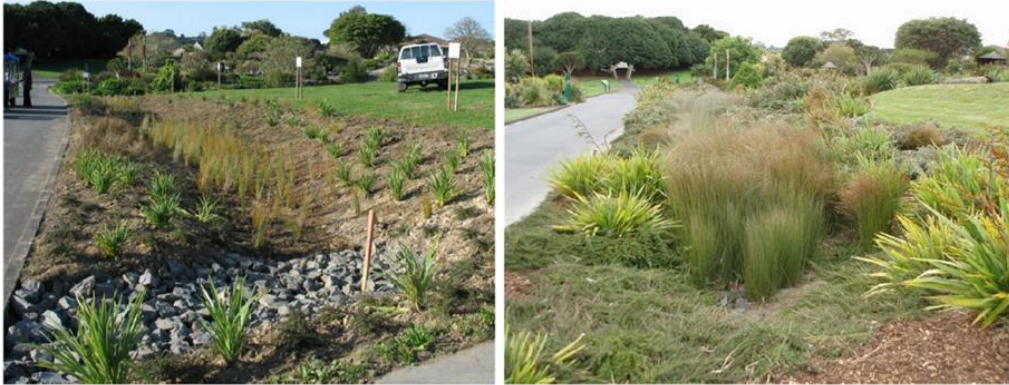
Bioretention swale about six months after planting and after about three years; plants on the well-drained edges are prostrate Coprosmas, prostrate manuka, mountain flax and scrambling pohuehue, with oioi in the wet base of the swale.
