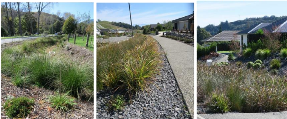
Nelson/Tasman Bioswale plantings. Left – stakes are used to allow fast identification for efficient weed control during establishment of this swale. Centre – a low-maintenance edge of gravel-mulched, short turutu ( Dianella nigra ) and taller oioi and knobby clubrush ( Ficinia nodosa ) in the centre. Right – Cyperus ustulatus in the centre of this raingarden is considered 'messy' by some people and may require removal of seed-heads to achieve suitable aesthetic outcomes in some localities.
