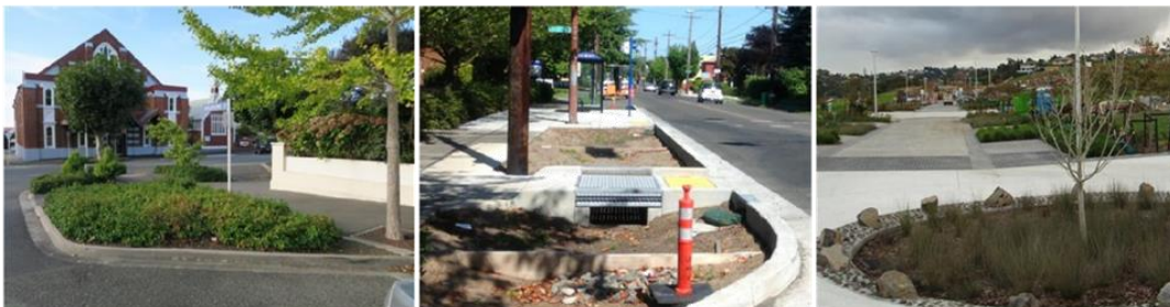
Bioretention can be located to provide multiple benefits: these three locations protect pedestrians from traffic, maintain clear views of intersections by preventing parking, and also receive the dirtiest runoff (corners are where brakes and tyres are worn, and spills are most likely to occur). Left – bump out in Nelson city could be converted to a raingarden; centre – bump out raingarden protects a bus stop and pedestrian crossing (Portland, Oregon, before planting); right – turn around raingarden with edges protected by boulders (North Harbour residential development).
