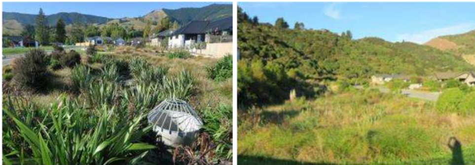
Examples of detention basins with healthy wetland plants in Tasman (left) and wetland in Nelson (right), 2017
