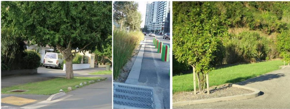
In the absence of a vertical 50 to 100 mm drop into a swale, physical barriers are usually important to exclude vehicles. Left – boulders used (Nelson); centre – bollards used (Melbourne); right – a clever use of curbs around trees (Nelson)
