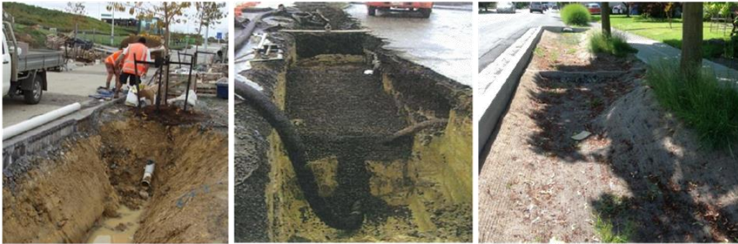
Left – placing trees between raingardens helps anchor trees and reduces damage to trees if raingardens are rejuvenated; the sloping sides at this site allow concrete retaining to be reduced. Right – bioretention swale showing underdrain and clean gravel drainage layer during construction. Deeper areas (foreground) support trees with 1000 mm media; between the trees the depth is 600 mm (photo by Chris Stumbles). Right – existing trees are incorporated into raingardens with a temporary cover of coir matting preventing weed establishment until planting.
