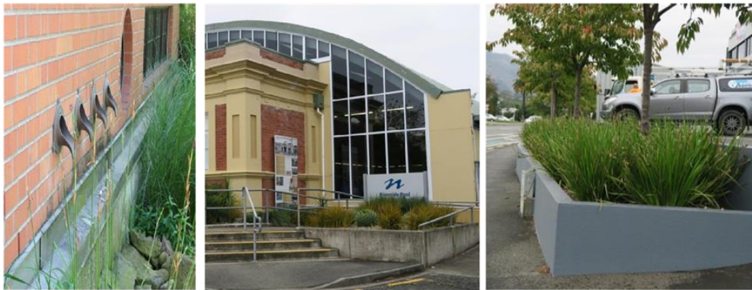
Stormwater planters and planter-possibilities: left – downpipe scuppers discharge onto rock-rip rap which removes energy from stormwater before it flows into planted bed; metal lining creates a hard-wearing edge against the building. Centre – This Nelson pool has planter boxes that could be easily re-purposed as planter boxes to capture runoff from the white downpipe. Right – Runoff from this Nelson carpark could be treated in the planter given suitable inlets and sub-drainage.
