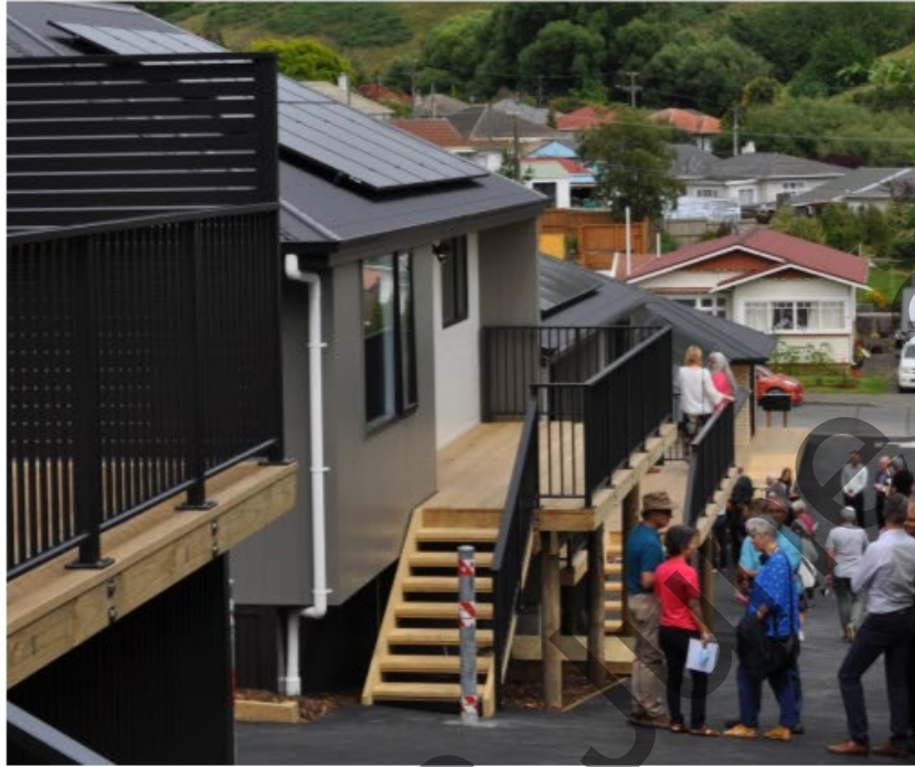
17 Murphy St, Toi Toi (at the Opening, 13 Dec 2021)
