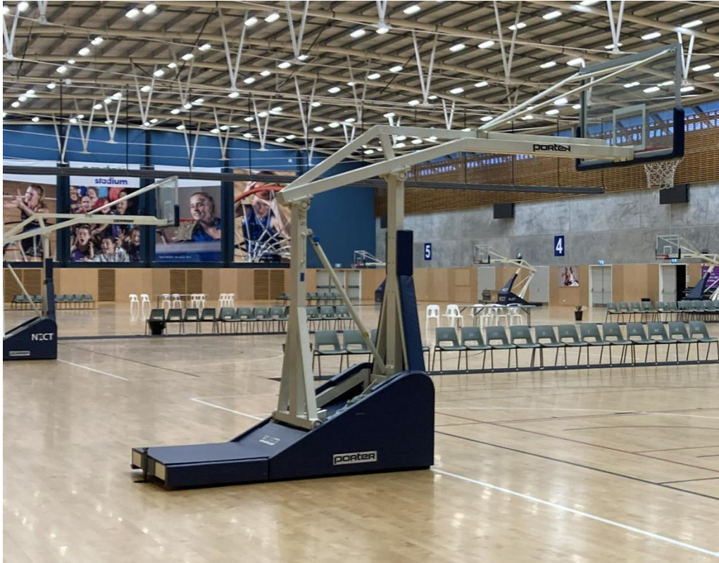
Figure 14 The floor-mounted basketball hoops at Saxton Field are reaching the end of their useful life and require renewal
