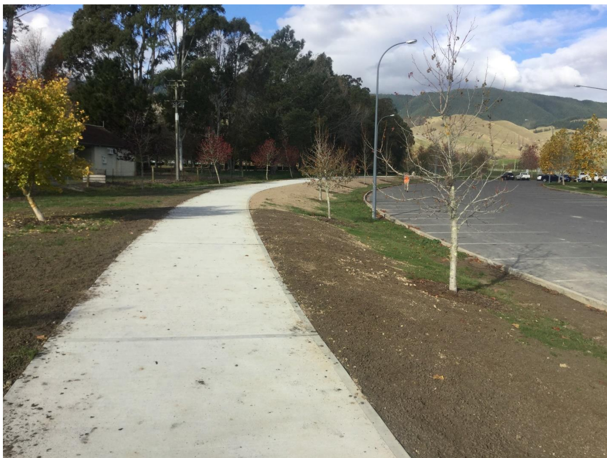
Figure 17 Completed new shared path north of Saxton Oval, 2022
