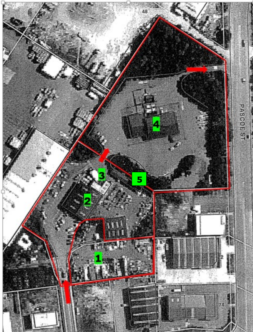
Figure 18: Aerial view of the Nelson Waste Recovery Centre
