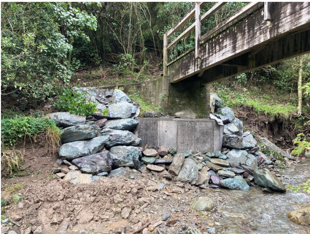
Figure 12: Barnicoat Track Bridge Abutment Repair, June 2023
