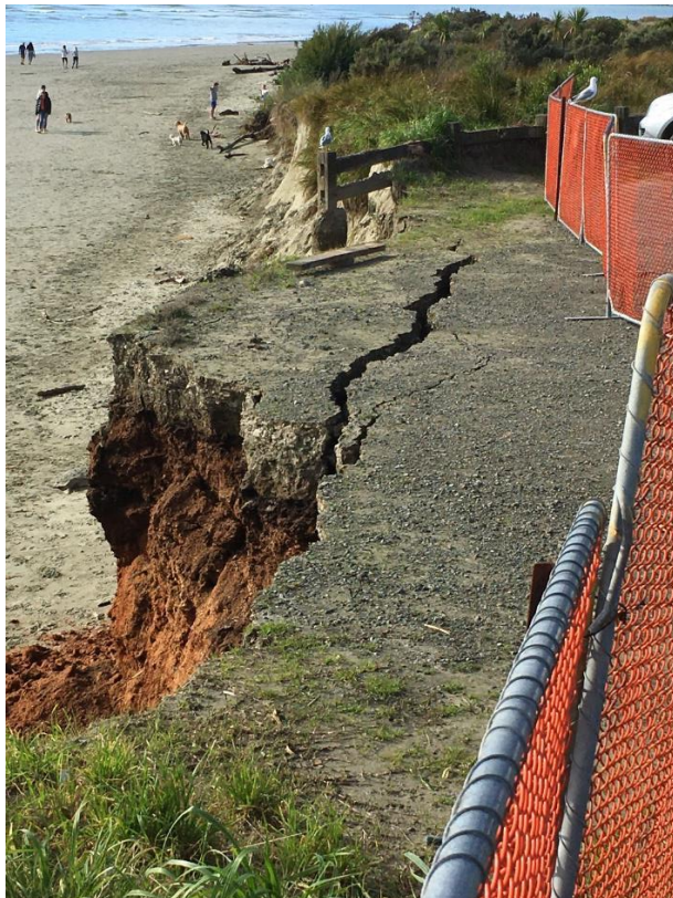
Figure 42: Erosion at Tāhunanui Back Beach, May 2023
