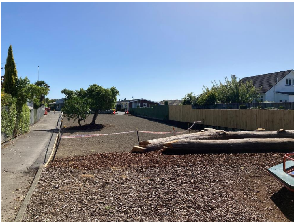
Figure 54: Development of newly acquired land (following house removal) that added important road frontage to Grove Reserve, March 2023
